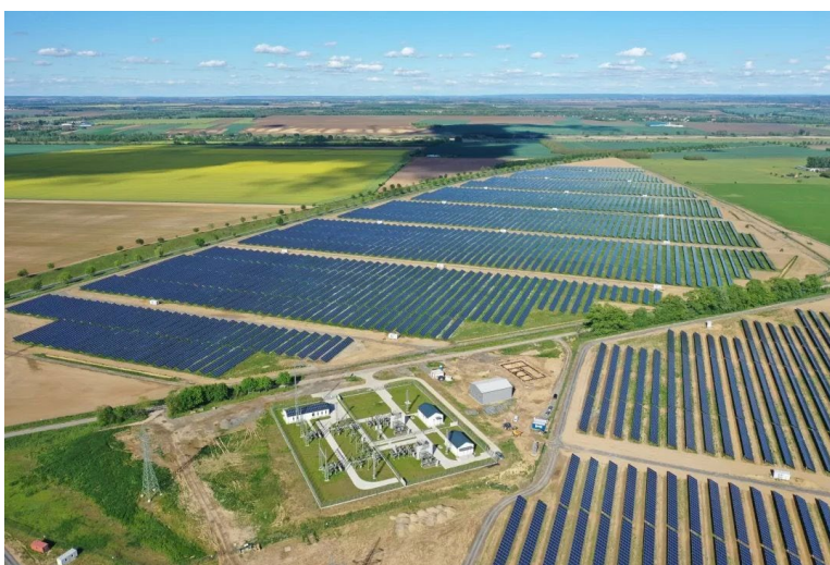
Aerial View of the Completed Power Plant, extracted from the official account of China General Technology Group in The Paper
