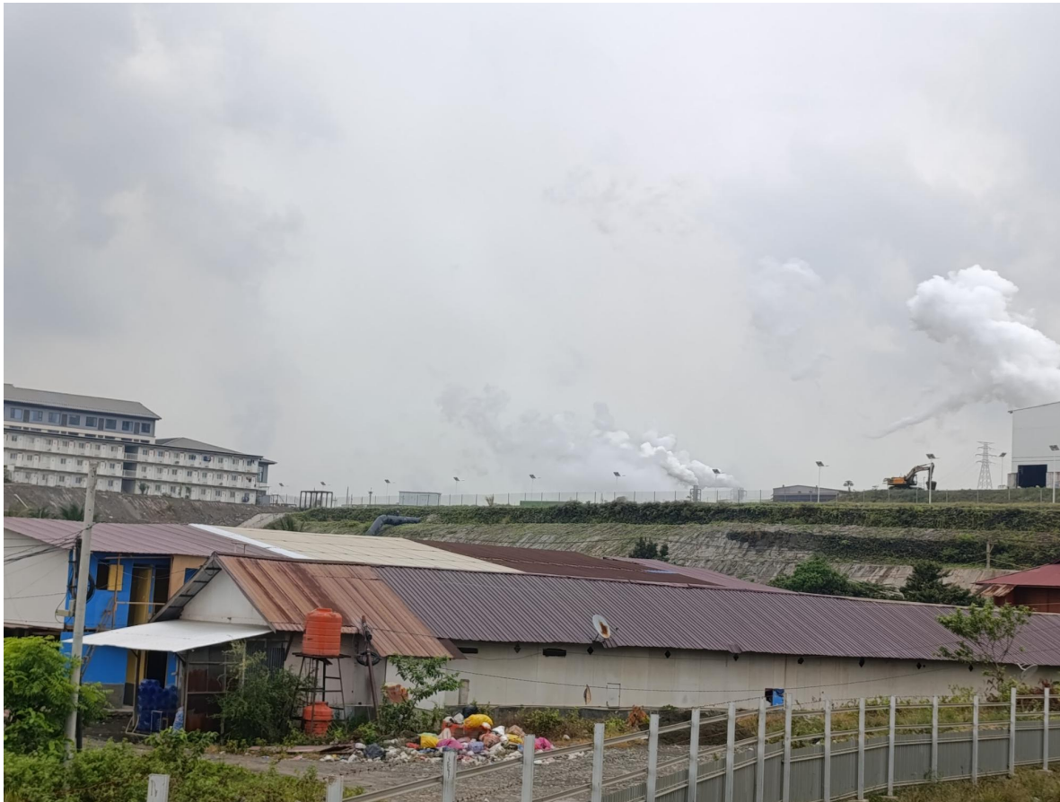
Figure 15 — Coal plant for nickel smelting, a joint venture of Jiangsu Delong Nickel Industry (currently in Administration), and Dexin Steel Indonesia (PTDSI), in Indonesia Morowali Industrial Park (IMIP); photo and text by Nursadah K , 6 October 2025
